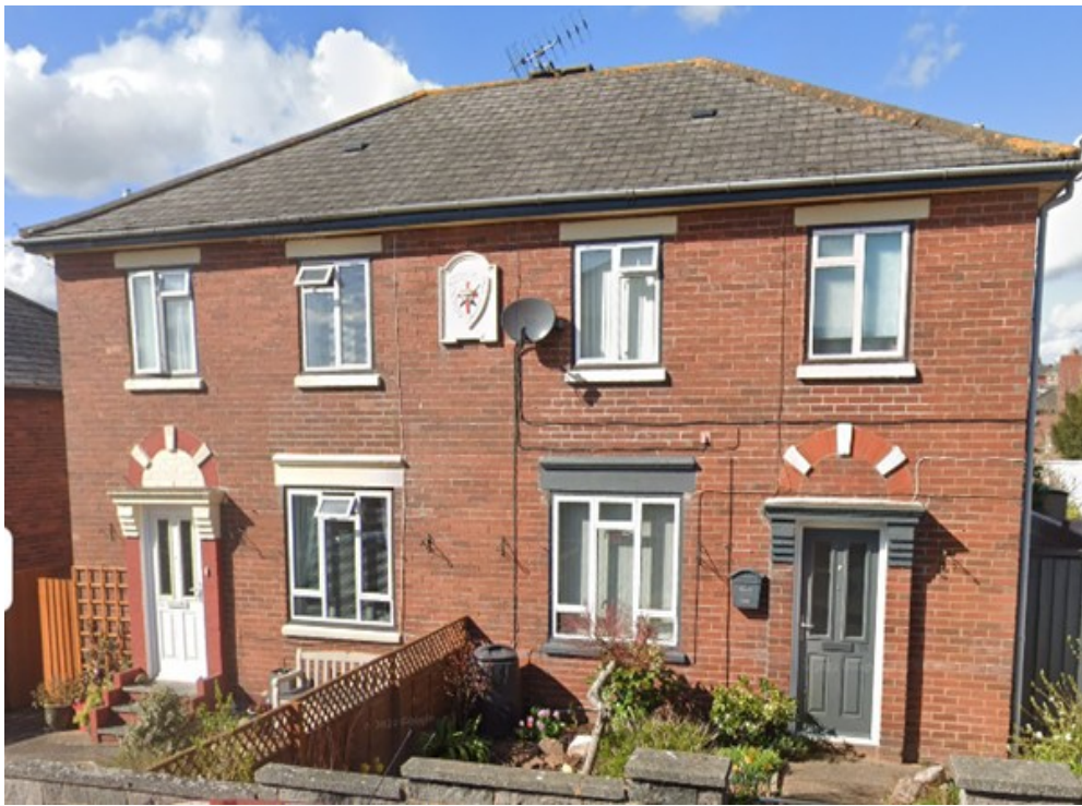
Rutherford Street Church Army Houses
