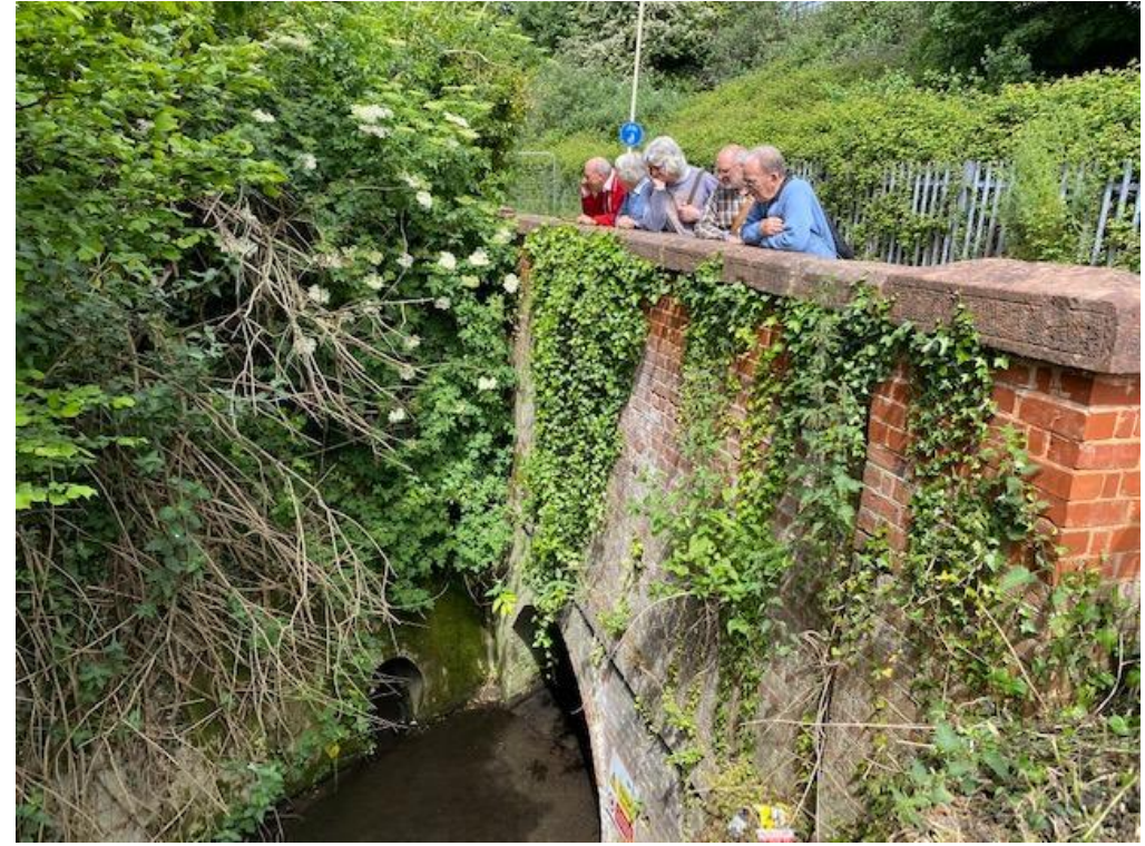
Northbrook emerging from its culvert by Polsloe Bridge station
